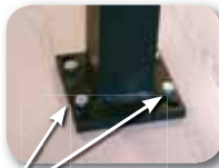
All Posts Self-Leveling w/Stainless Steel Shims
